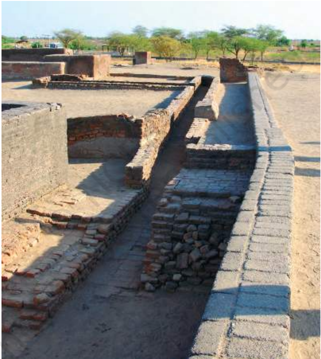
Fig. 6.7. Drainage system at Lothal (Gujarat)
