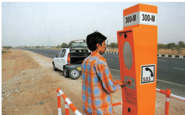
Fig. 7.10 : Emergency call box on NH-48
