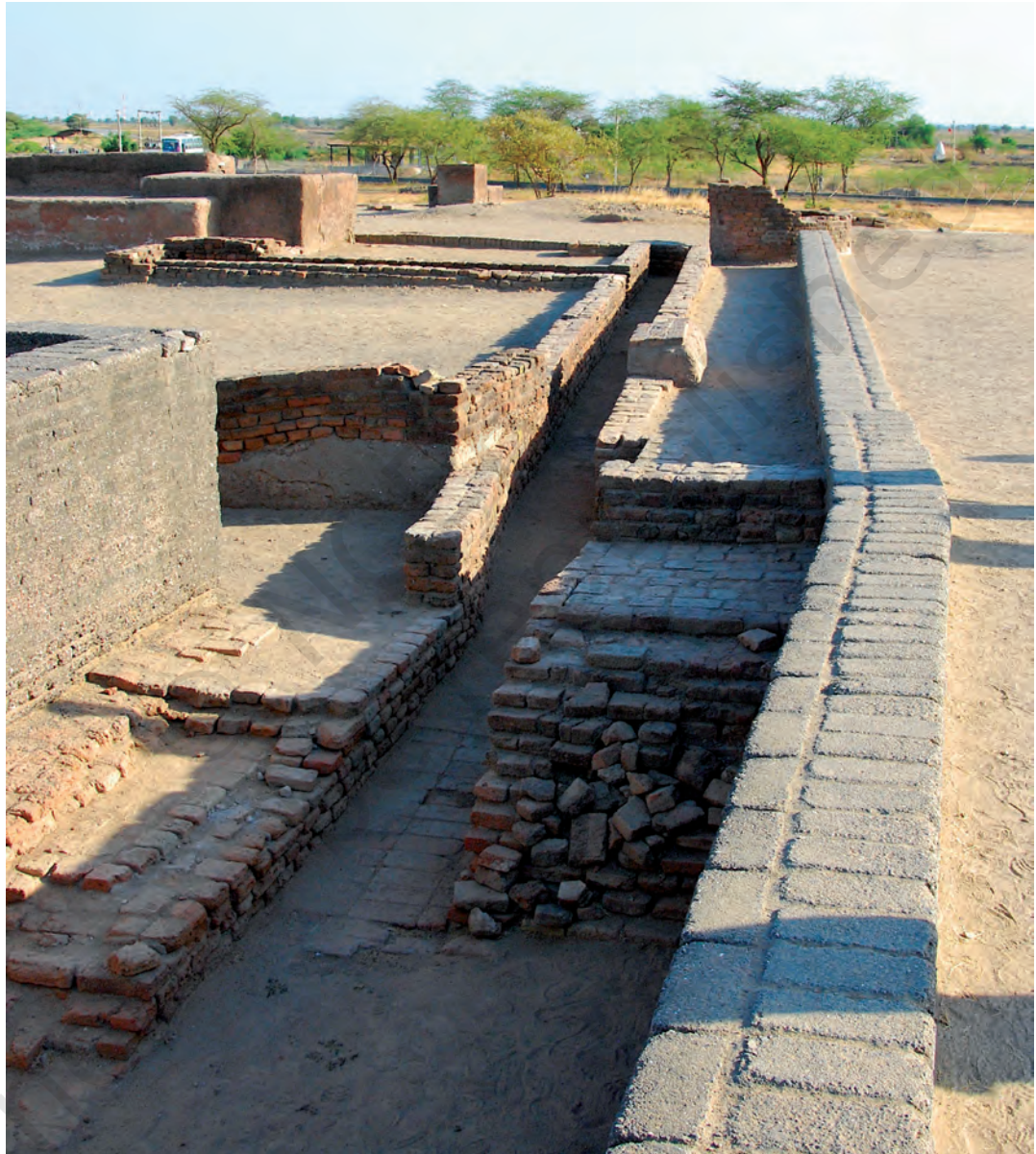
Fig. 6.7. Drainage system at Lothal (Gujarat)
